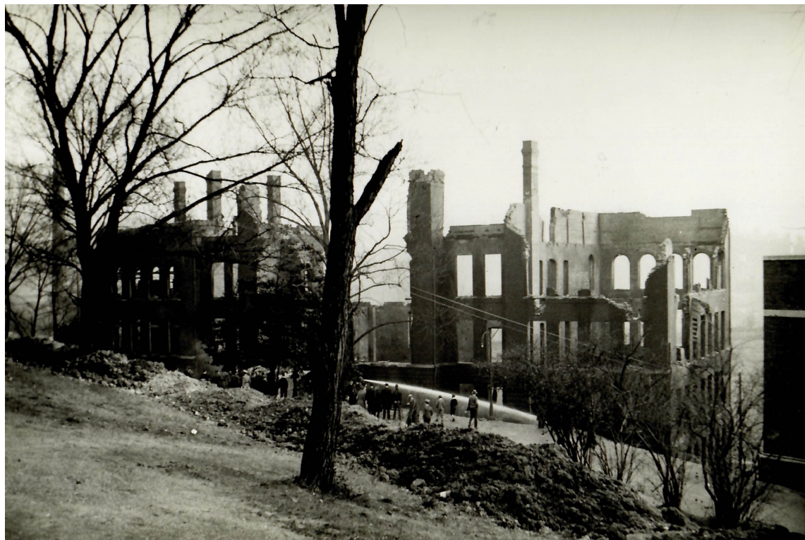
Fig. 2. Morrill Hall after the fire, January 1934. Courtesy of the TENN herbarium.
